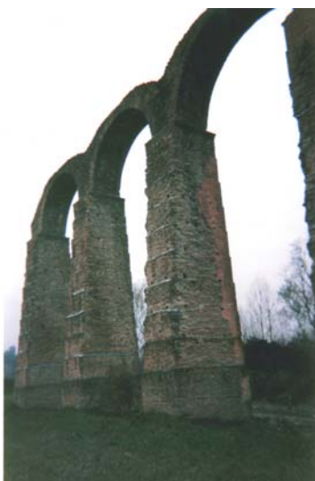
Stone masonry, Aquis Terme, Italy
