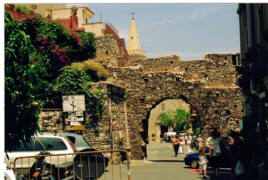
Brick and stone layers masonry, Taormina, Italy
