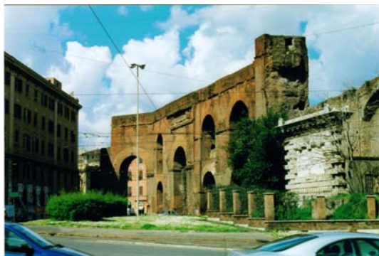
Brick faced concrete, Nero's branch, Rome
