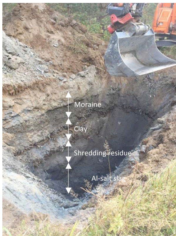
Figure 4: Landfill layers at the Vierumäki industrial landfill.
