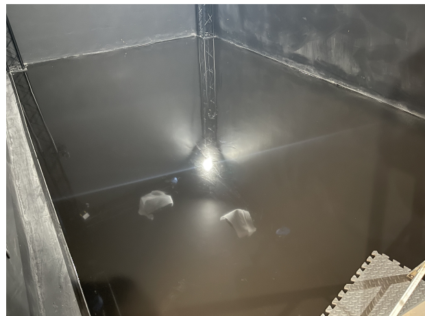
Figure 5: LAND EPOXY floor
