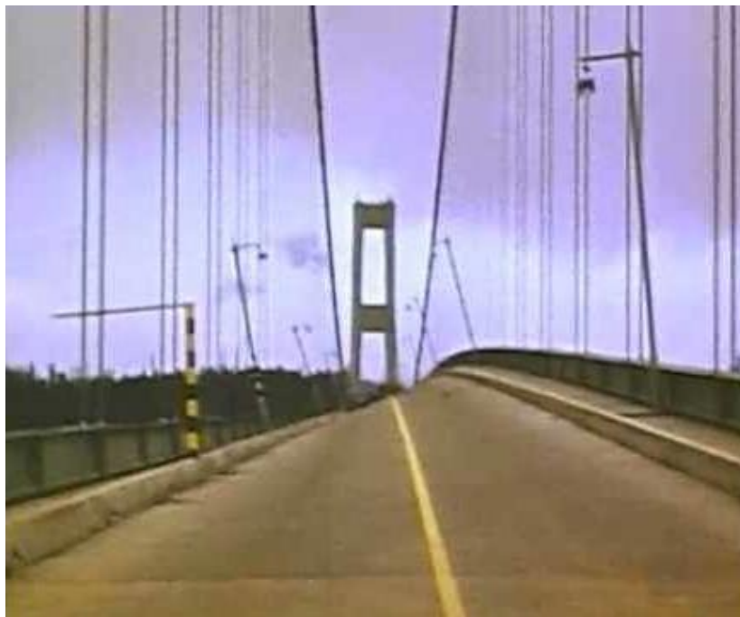
Figure 1 Tacoma Narrows bridge twisting, allthatsinteresting
