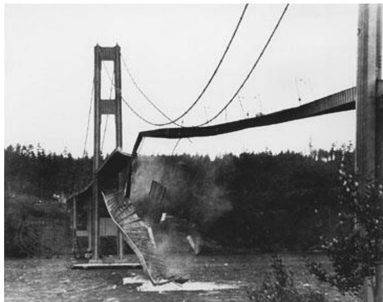
Figure 2 Tacoma Narrows bridge collapse, allthatsinteresting
