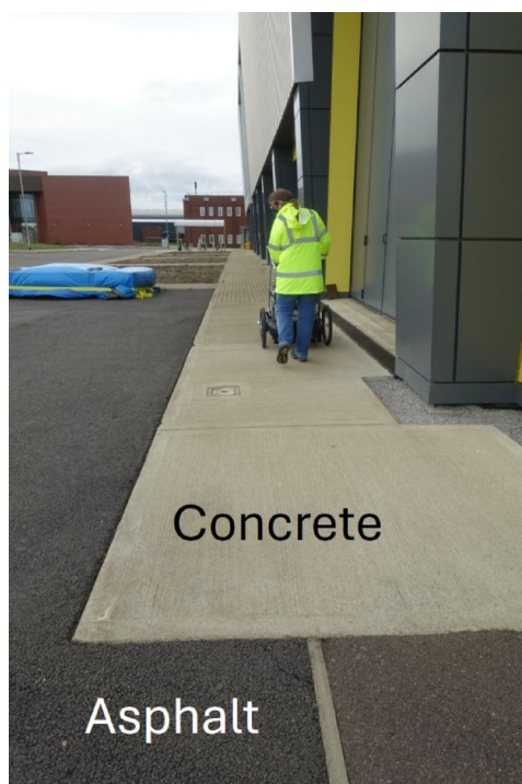
Fig. 23. Photograph of location used to make measurements of instrument response to change in surface material (asphalt to concrete).
