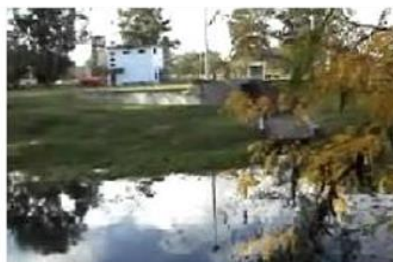
C2: Fray Bentos stream at wastewater discharge
