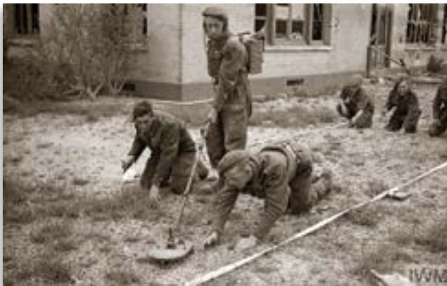
An older model Polish mine detector (PMD) being used to search the grounds of a hotel in Luc-Sur-Mer, Normandy, July 1944. PMDs gave good service but struggled against low metal content mines or, as for modern EMI detectors, in areas of metal contamination. Note the lack of safety distances or personal protective equipment employed. Image IWM B 7342.
