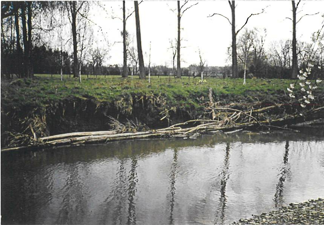
Plate 3 River Arrow, April 1993, post-maintenance
