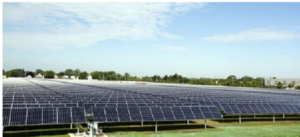
Figure 6.1. SunPower PV panels mounted in single-axis tracker systems in Exelon City Solar (Source: SolarServer)
