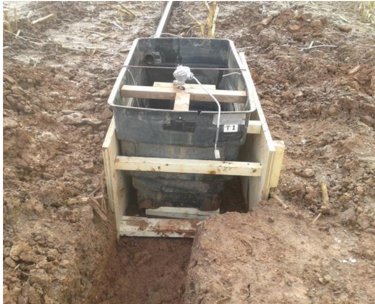
Figure 5 Particular the stabilisation of a tank during Experiment 1.
