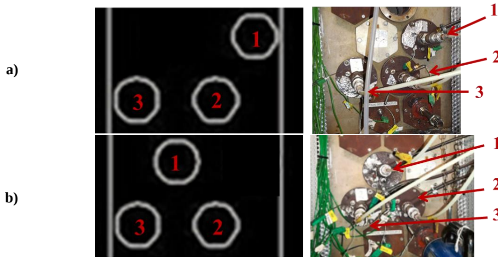
Figure 6-1: Configuration of the air cooled ceramic probes during combustion of pulverised Daw Mill-12 wt.% Miscanthus in Cranfield's combustion rig: a) first configuration; b) second configuration.
