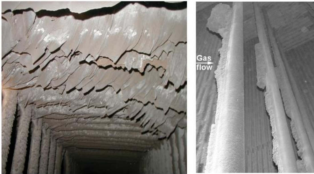
Figure 2-6: Ash slagging (left) (Mengenai, 2014); deposit fins on superheater tubes (right) (Tomeczek et al., 2004).
