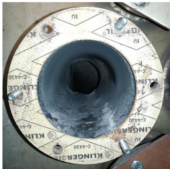
Figure 5-29: Ash collection from one of the ports along the vertical section of the combustor used to place the probe.
