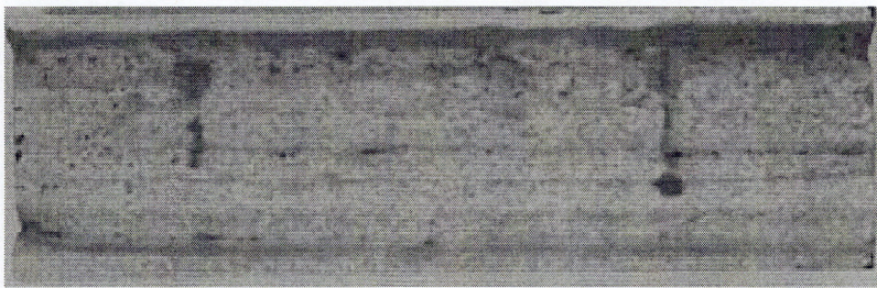
Figure 92: IIIS1MO325 – Die penetrant inspection after welding.
