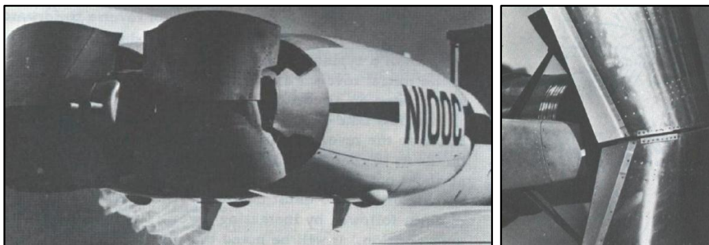
Figure 3.36: (L) Dual target reverser, Lockheed Jet star business jet. (R) Target thrust reverser on Grumman Gulfstream II business jet. Images adopted from [Ref. 33]
